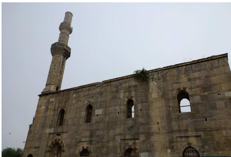
Picture 15. Vajazit Mosque
